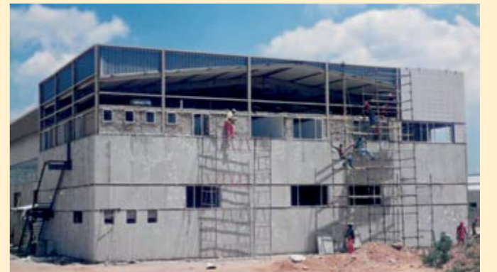
1997 PMSA under construction in Honeydew
