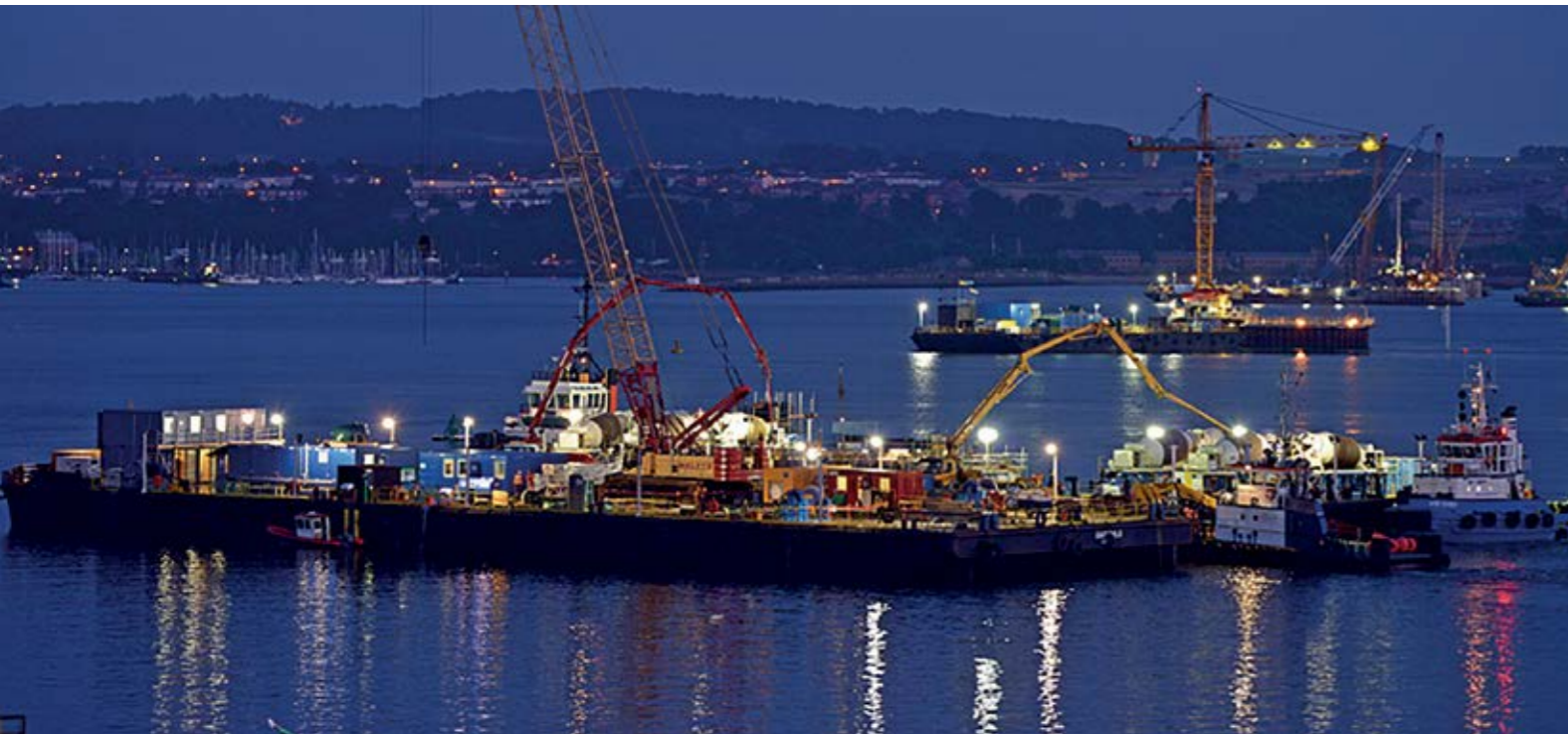
▲ The day passes...the concrete pump arrives: Concrete was poured around the clock for 15 days at the south pillar of the Firth of Forth bridge.
