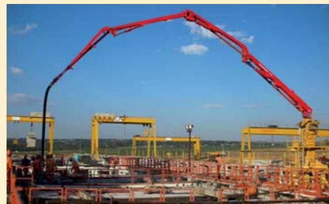
2007 MX 24 at the Precast yard for the Gautrain project
