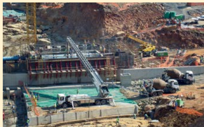
2007 A Telebelt TB 130 was used for the hydropower scheme in Lady-Smith, Kwa-Zulu Natal Province
