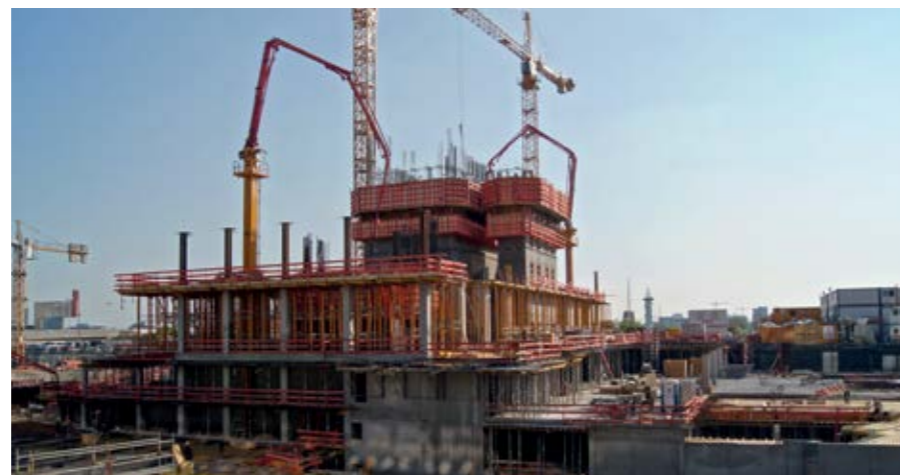
▲ Construction site for the DC Tower in Vienna in spring 2011
