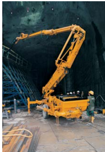
▲ Tunnel puma in use at the Goldisthal pump storage works (2000)
