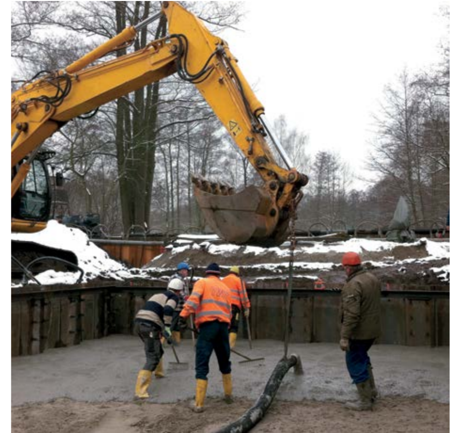
◀▲ The concrete for the sluice floor is distributed using flexible delivery hoses and excavators.
