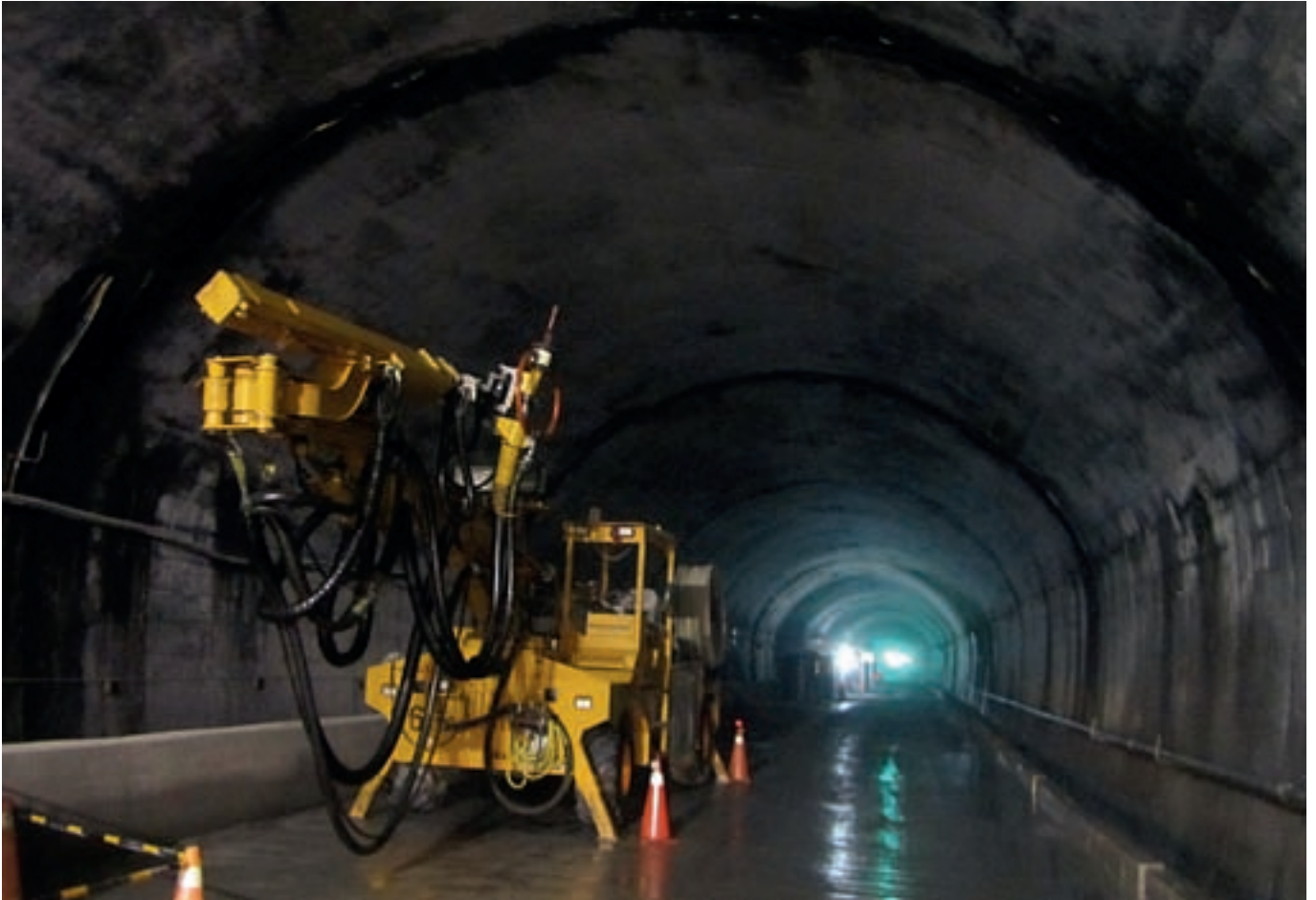
▲ One of the twelve SPM 500 Wetkret inside the tunnel
