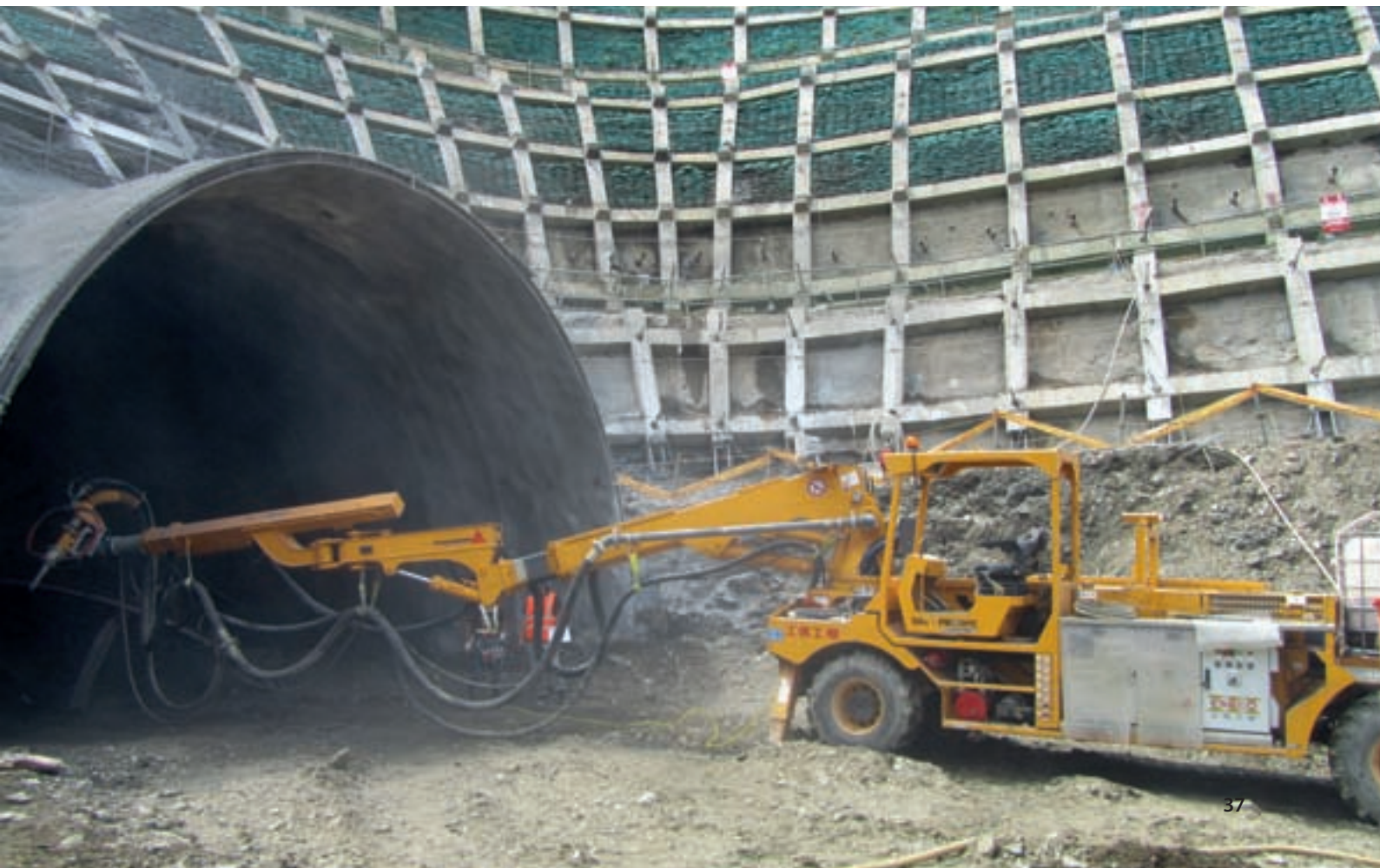
▼ A SPM 500 Wetkret on one of the tunnel portals
